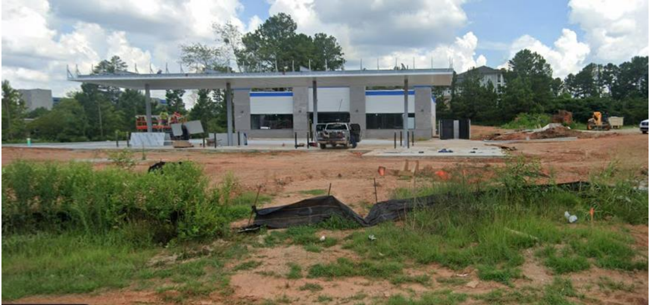
Figure 1: AAA22-000002 6030 Hillandale Drive
