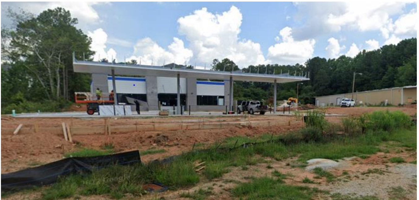
Figure 2: AAA22-000002 6030 Hillandale Drive
